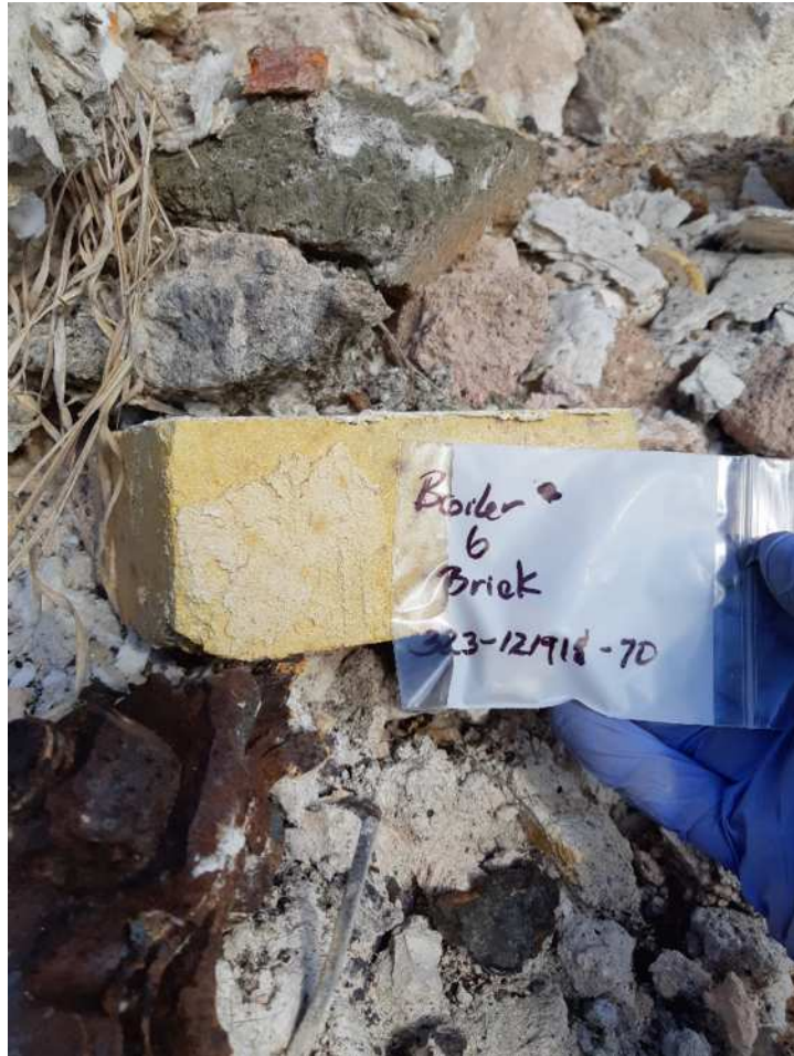
General View Sample # 70, Boiler #6, Inside Brick.
