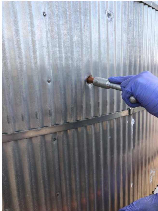
General View Sampling Point #19, TSI Tower #6, Northeast Side.
