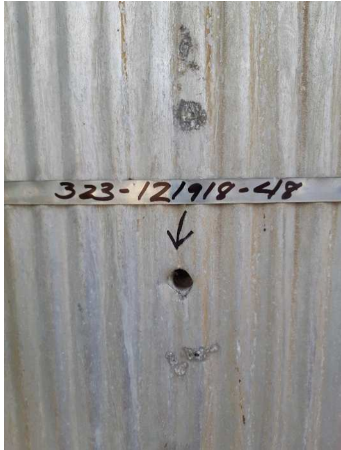
General View Sampling Point #48, Tower 11 TSI, Northeast Side.
