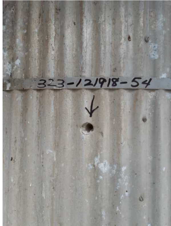
General View Sampling Point #54, Tower 12, South Side
