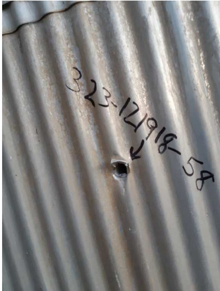
General View Sampling Point #58, Tower 13, West Side
