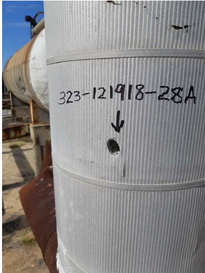
General View Sampling Point #28A, Tank 2, 10' \varnothing TSI, East Side.
