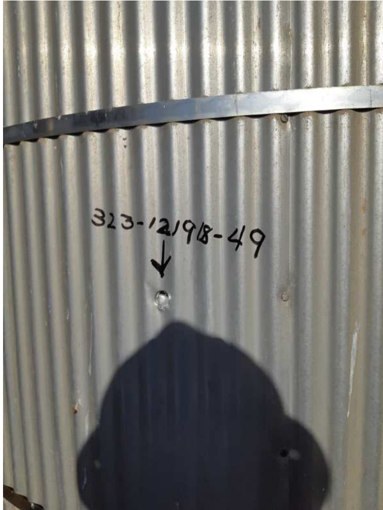
General View Sampling Point #49, Tower 11 TSI, South Side.
