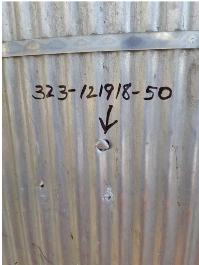
General View Sampling Point #50, Tower 11 TSI, North Side.
