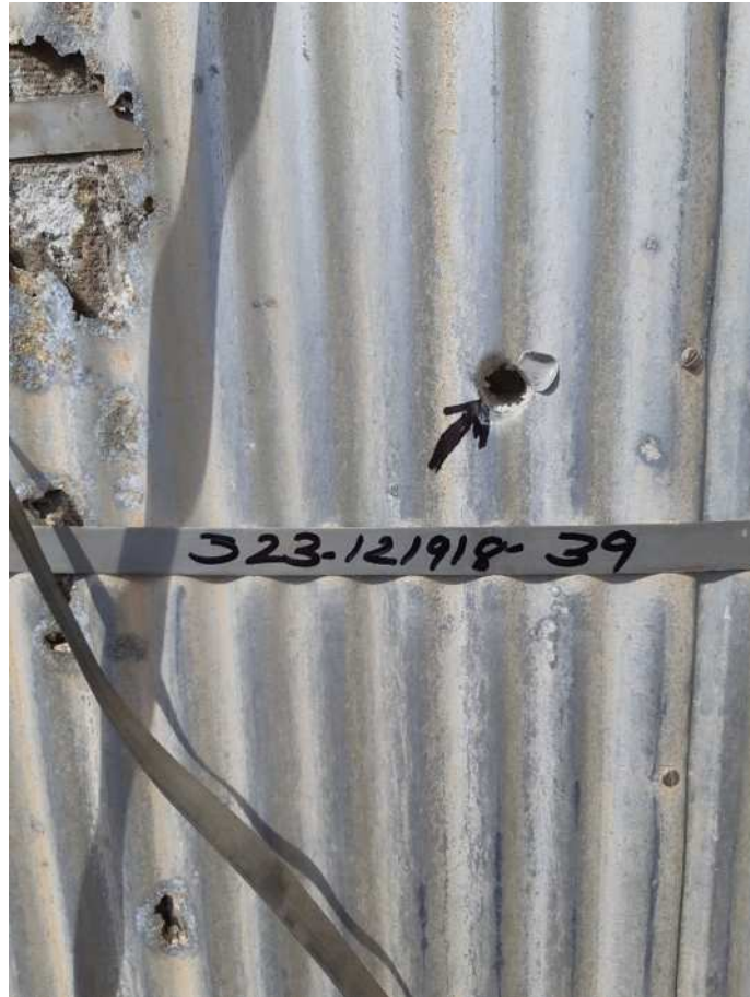
General View Sampling Point #39, Tank 6 TSI, South Side.
