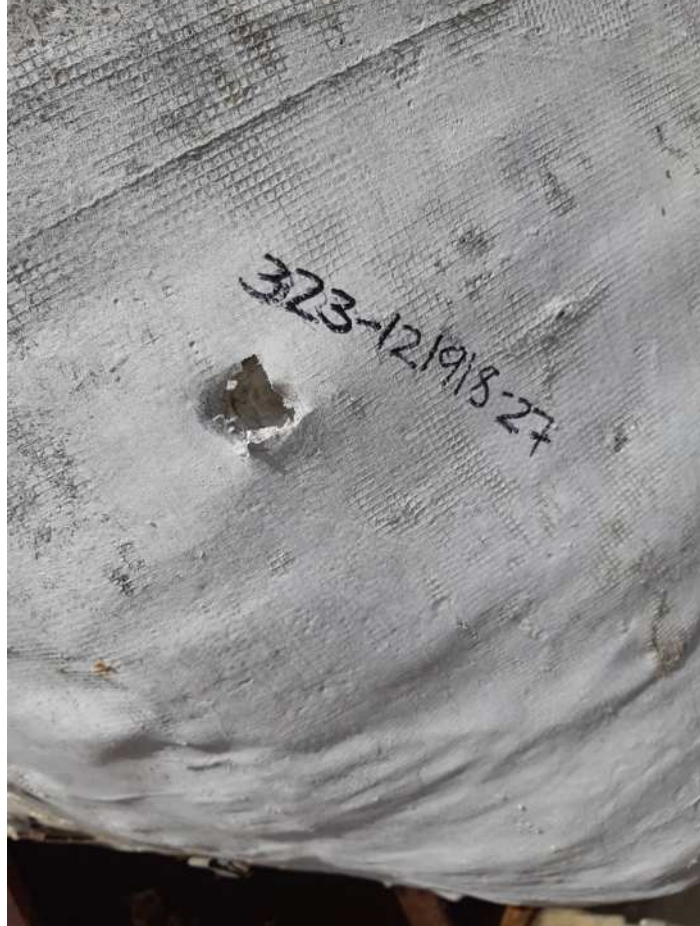
General View Sampling Point #27, Tank 2 TSI, North Side.
