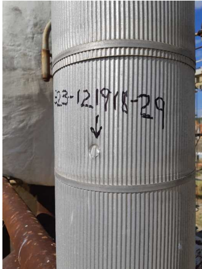
General View Sampling Point #29, Tank 2 TSI, South Side.
