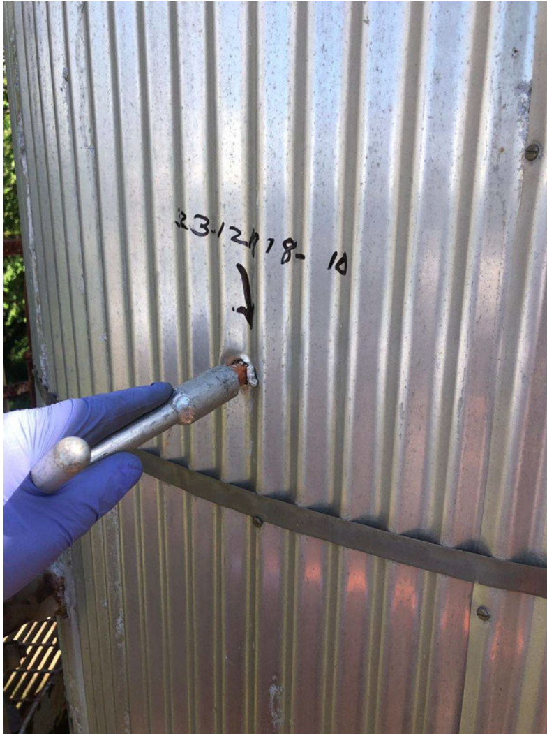
General View Sampling Point #10, TSI Tower #3, South Side
