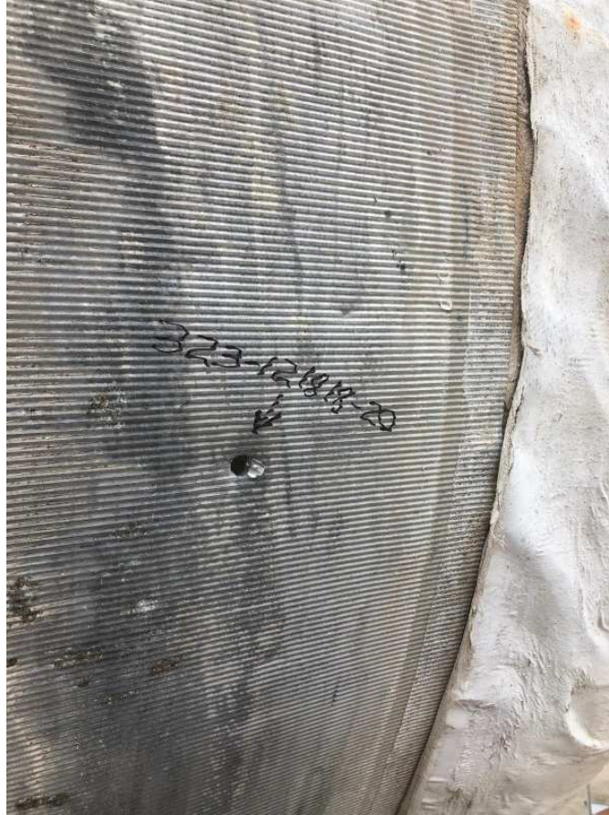
General View Sampling Point #20, TSI Tower #6, South Side.
