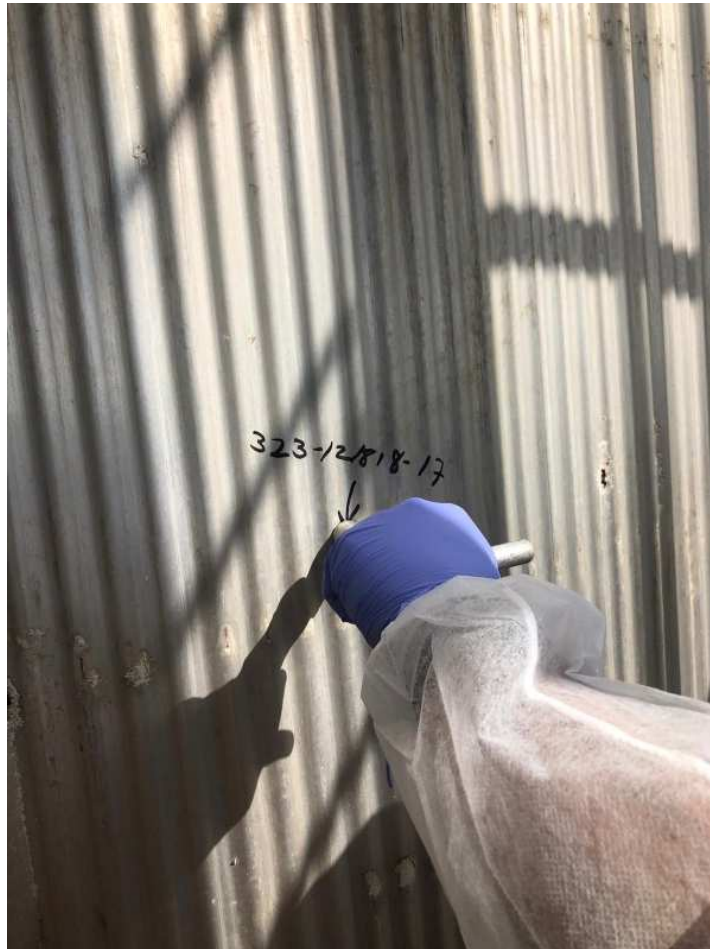
General View Sampling Point #15, TSI Tower #5, South Side.
