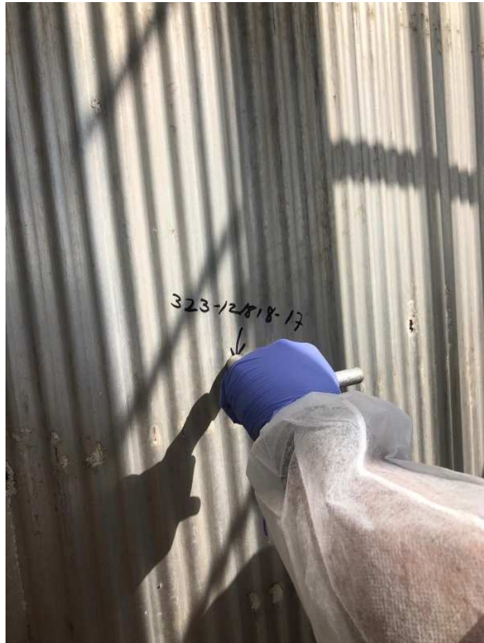
General View Sampling Point #17, TSI Tower #6, South Side.
