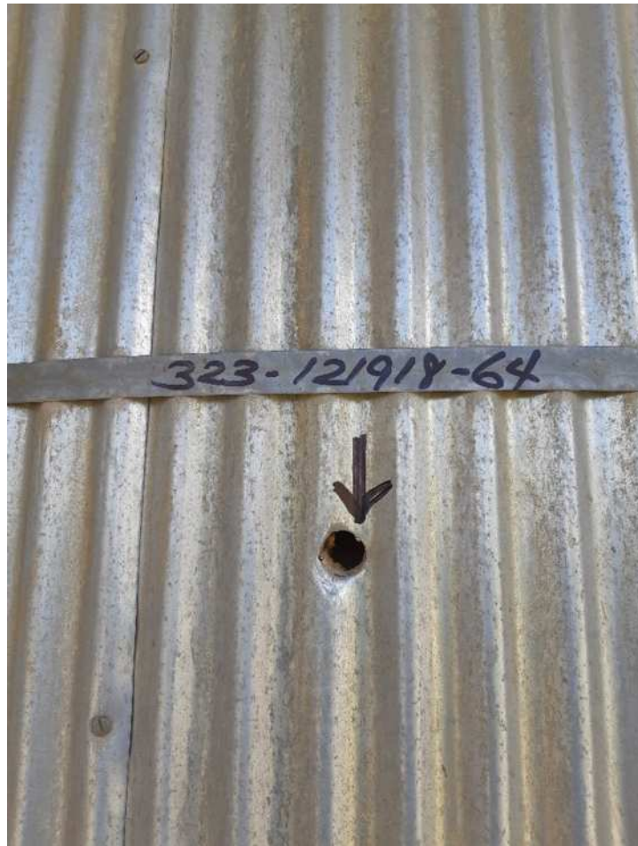
General View Sampling Point #64, Tank 7, Northeast Side
