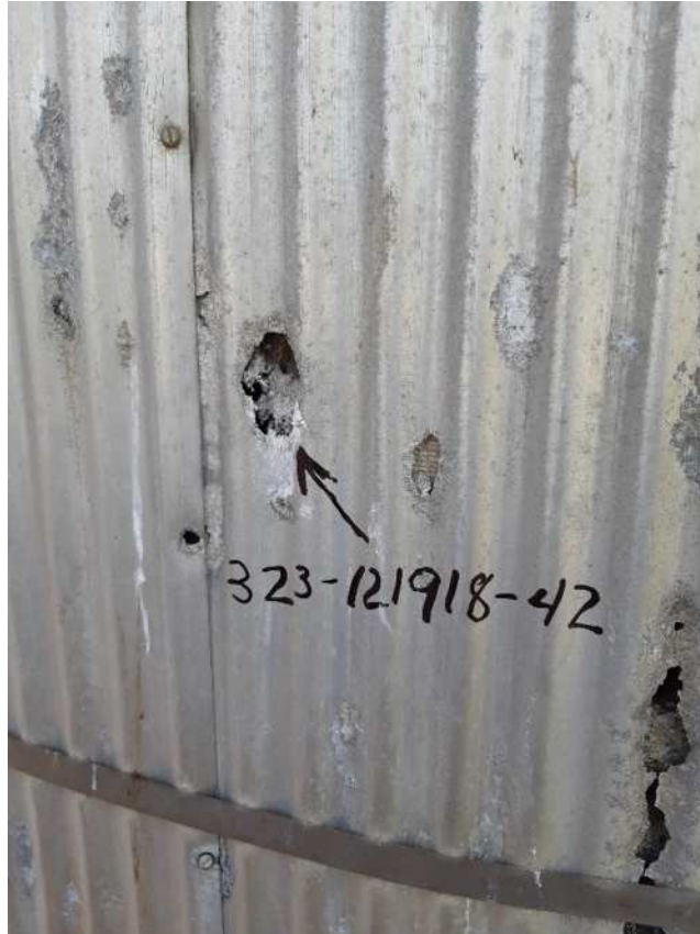
General View Sampling Point #42, Tower 9 TSI, South Side.
