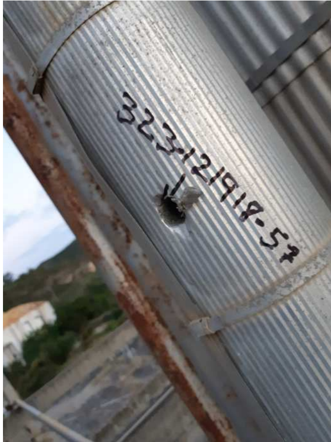
General View Sampling Point #57, TSI 6'ø, Tower 13, North Side
