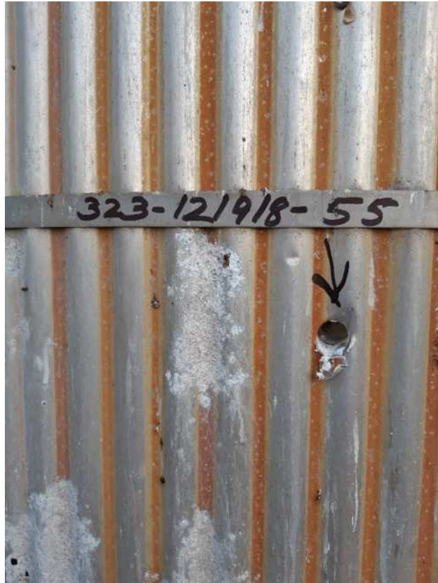
General View Sampling Point #55, Tower 12, North Side
