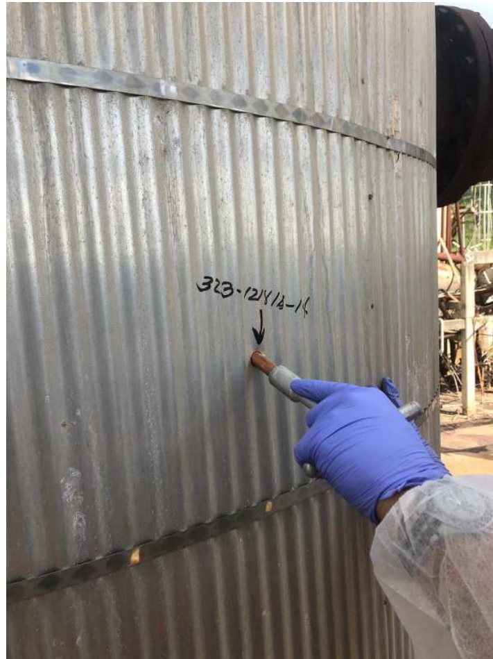
General View Sampling Point #14, TSI Tower #4, Southwest Side.
