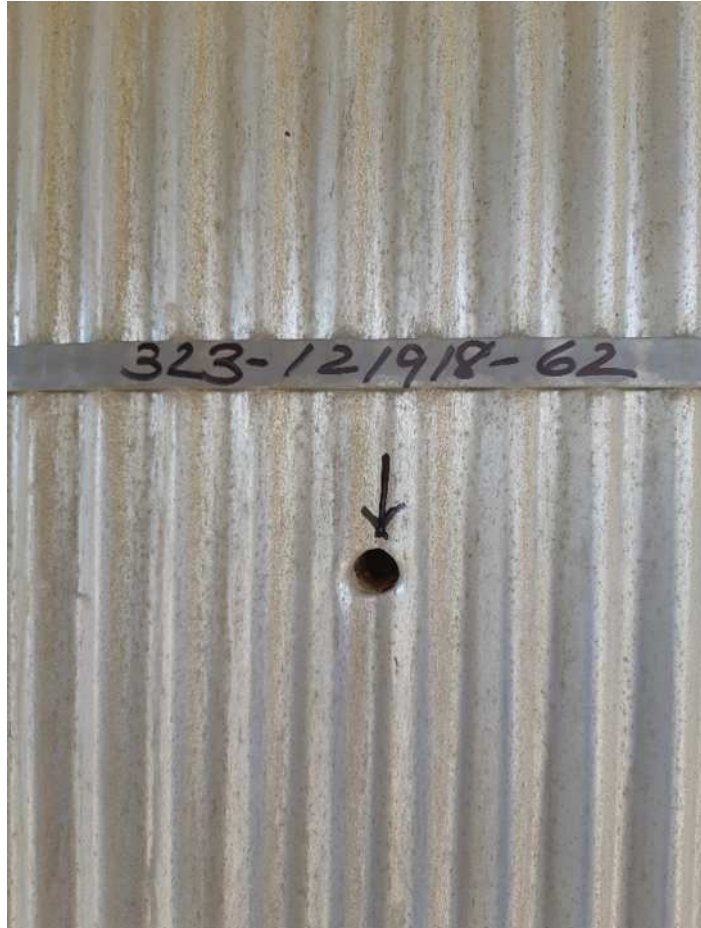
General View Sampling Point #62, Tank 6, Northeast Side
