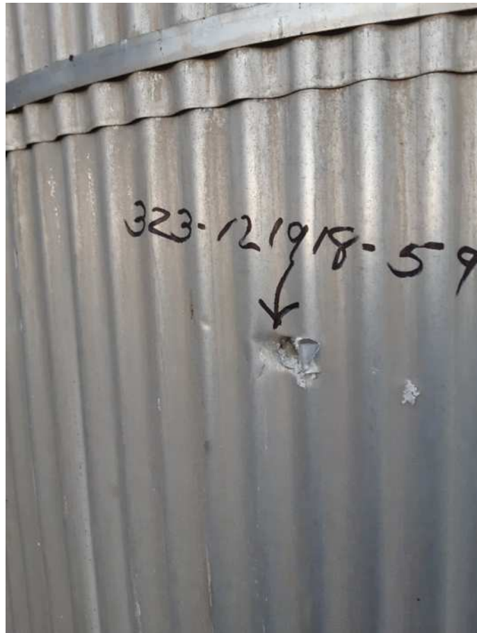
General View Sampling Point #59, Tower 13, South Side
