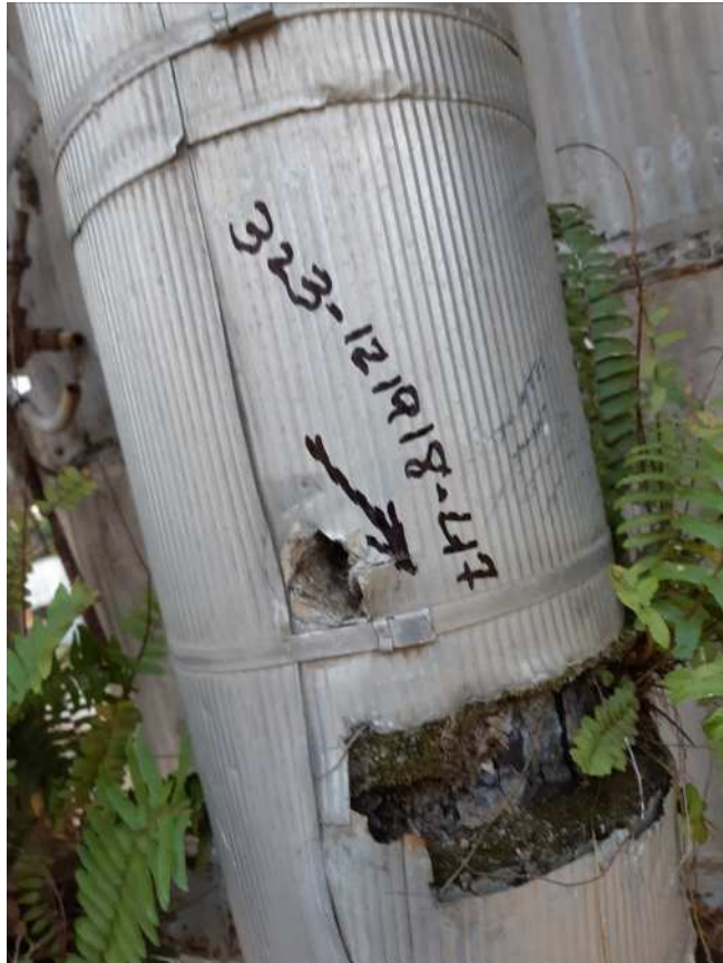
General View Sampling Point #47, 8'' \phi Pipe, Tower 10 TSI, Northeast Side.
