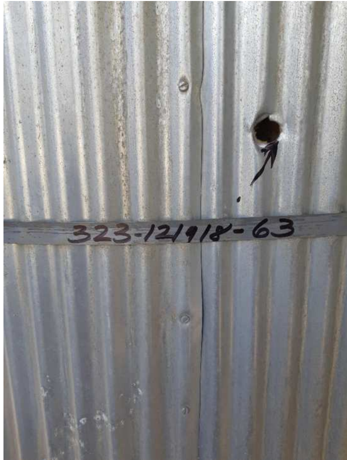
General View Sampling Point #63, Tank 6, North Side
