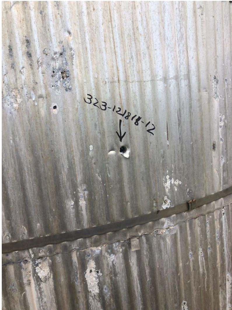
General View Sampling Point #12, TSI Tower #4, South Side
