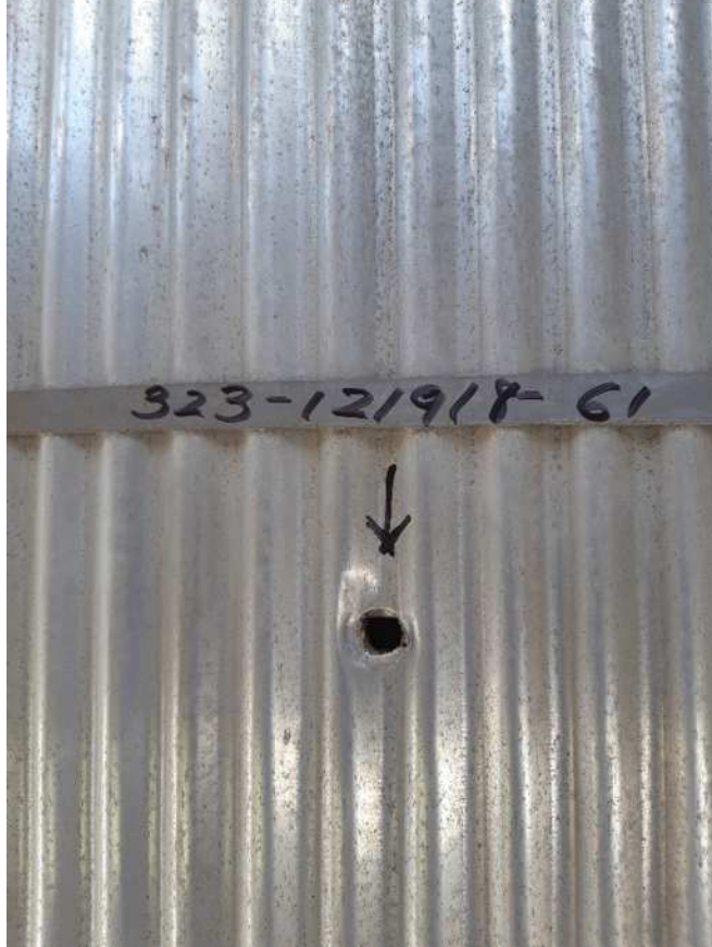
General View Sampling Point #61, Tank 5, North Side
