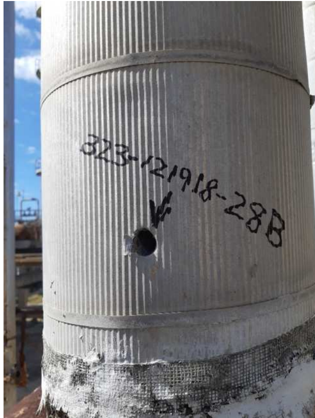
General View Sampling Point #28B, Tank 2, 10' \phi TSI, East Side.
