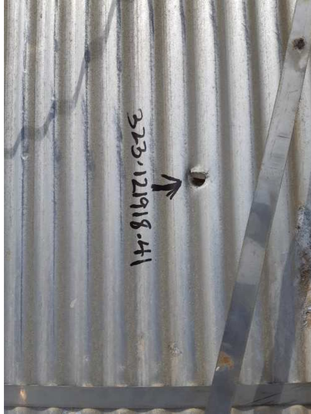
General View Sampling Point #41, Tank 6 TSI, North Side.
