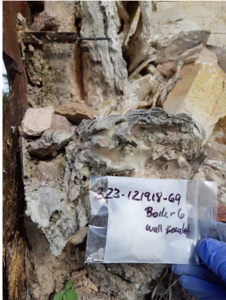
General View Sample # 69, Boiler #6, Inside Insulation Wall(white).
