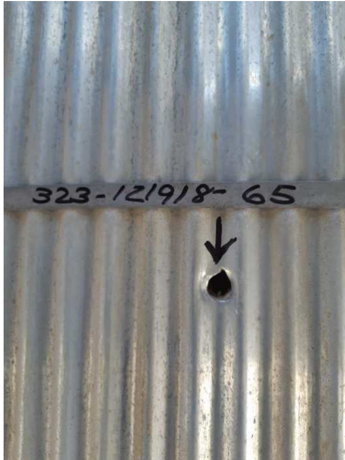
General View Sampling Point #65, Tank 7, North Side
