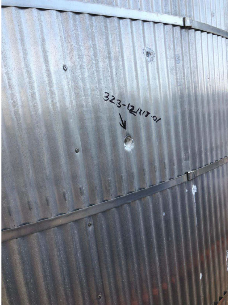
General View Sampling Point #1, TSI Tower #1 South Side
