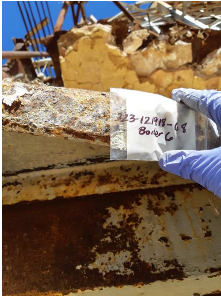
General View Sample # 68, Boiler #6, Fireproofing Cloth Between Metal Walls
