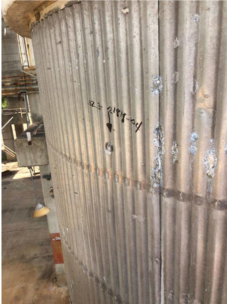
General View Sampling Point #4, TSI Tower #2 South Side
