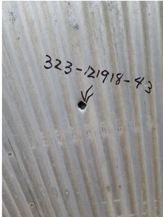
General View Sampling Point #43, Tower 9 TSI, North Side.
