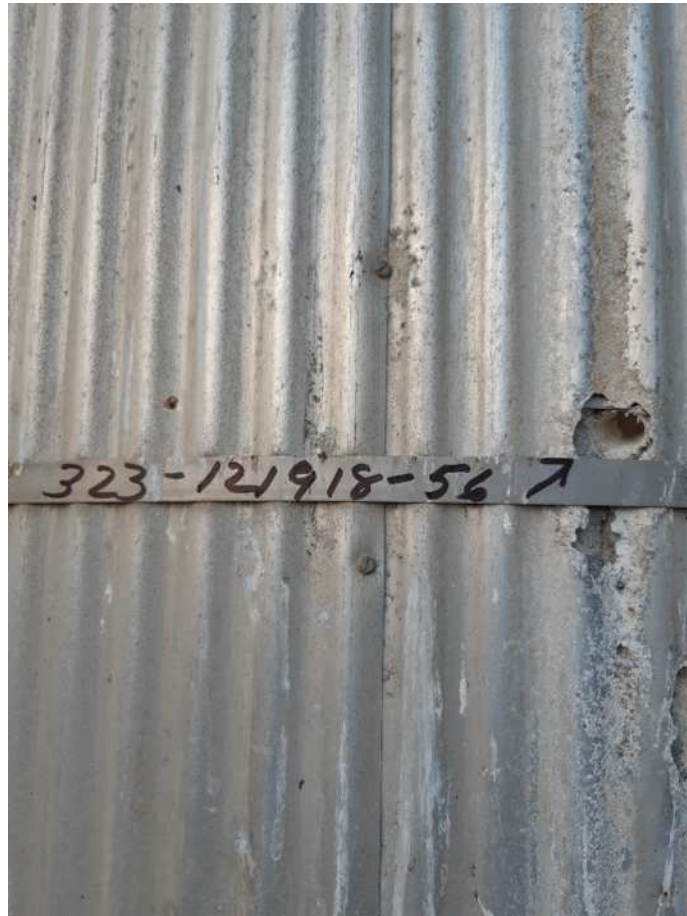
General View Sampling Point #56, Tower 12, West Side
